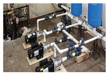
In 2017, the museum began its plan to improve the quality of water by connecting to the municipal water main line supply. In May of 2020, the boost pumps installed in the fall of 2019 went online as a means to providing adequate water pressure around the grounds and public campground.
